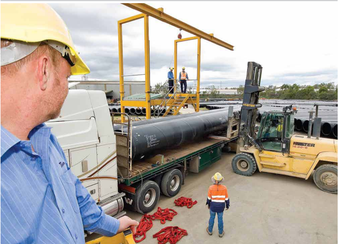
Loading DN1000 SINTAKOTE steel pipe
