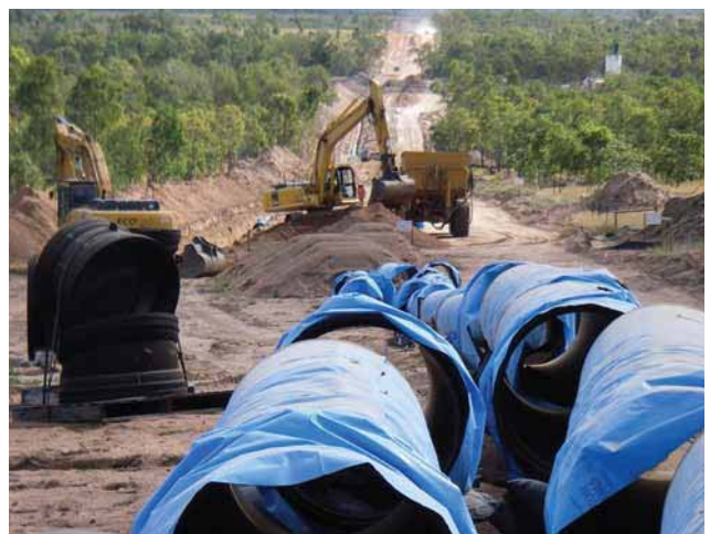
Corrosion Protection – Blueboss, loose polyethylene sleeving
