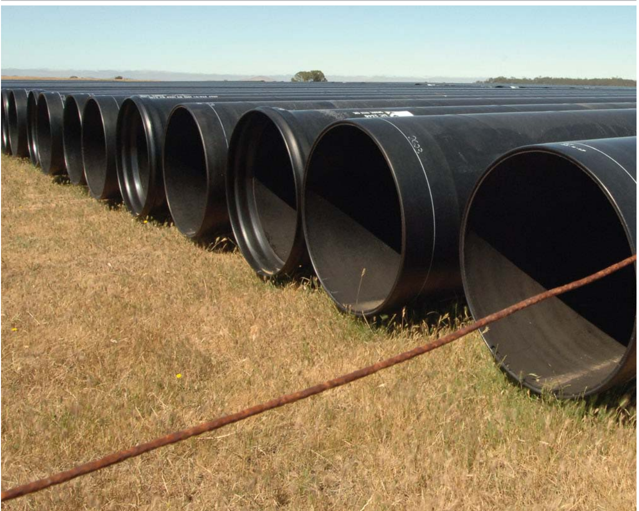
SINTAKOTE steel pipes awaiting installation on the Bendigo to Ballarat pipeline
