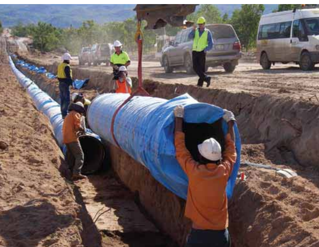
Installing DN600 Ductile Iron pipe
