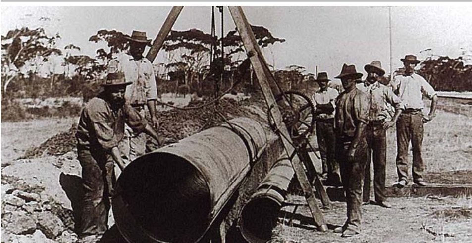
Golden Pipeline installation techniques
